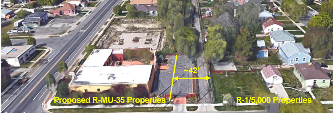
The above image shows the effective rear setback that would be required by the proposed R-MU-35 zone.
